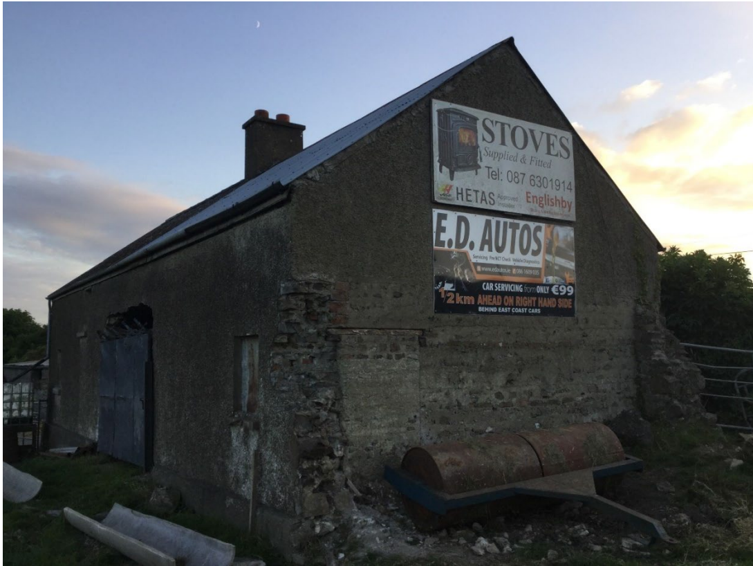
Plate 1. View from the north eastern side of Building A
