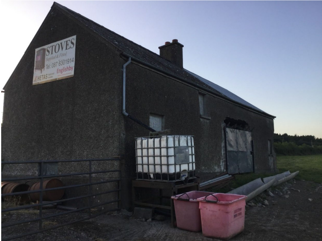
Plate 3. View from the south eastern side of Building A
