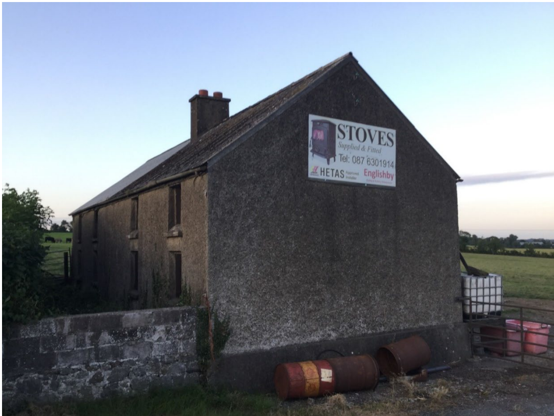
Plate 2. View from the south western side of Building A
