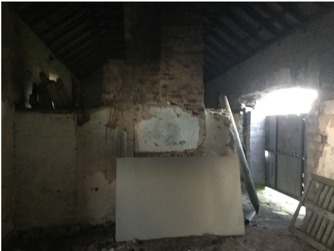
Plate 4. View from the interior of Building A showing chimney
